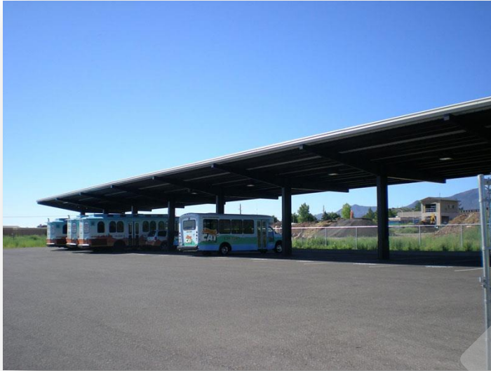
Figure 3.3 Outdoor covered storage
