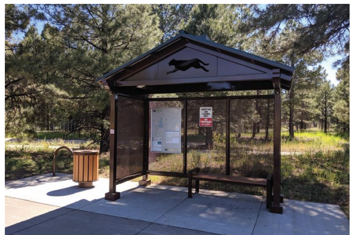
Type III bus stop in Flagstaff with bike rack, trash can, shelter, landing pad and signage.
