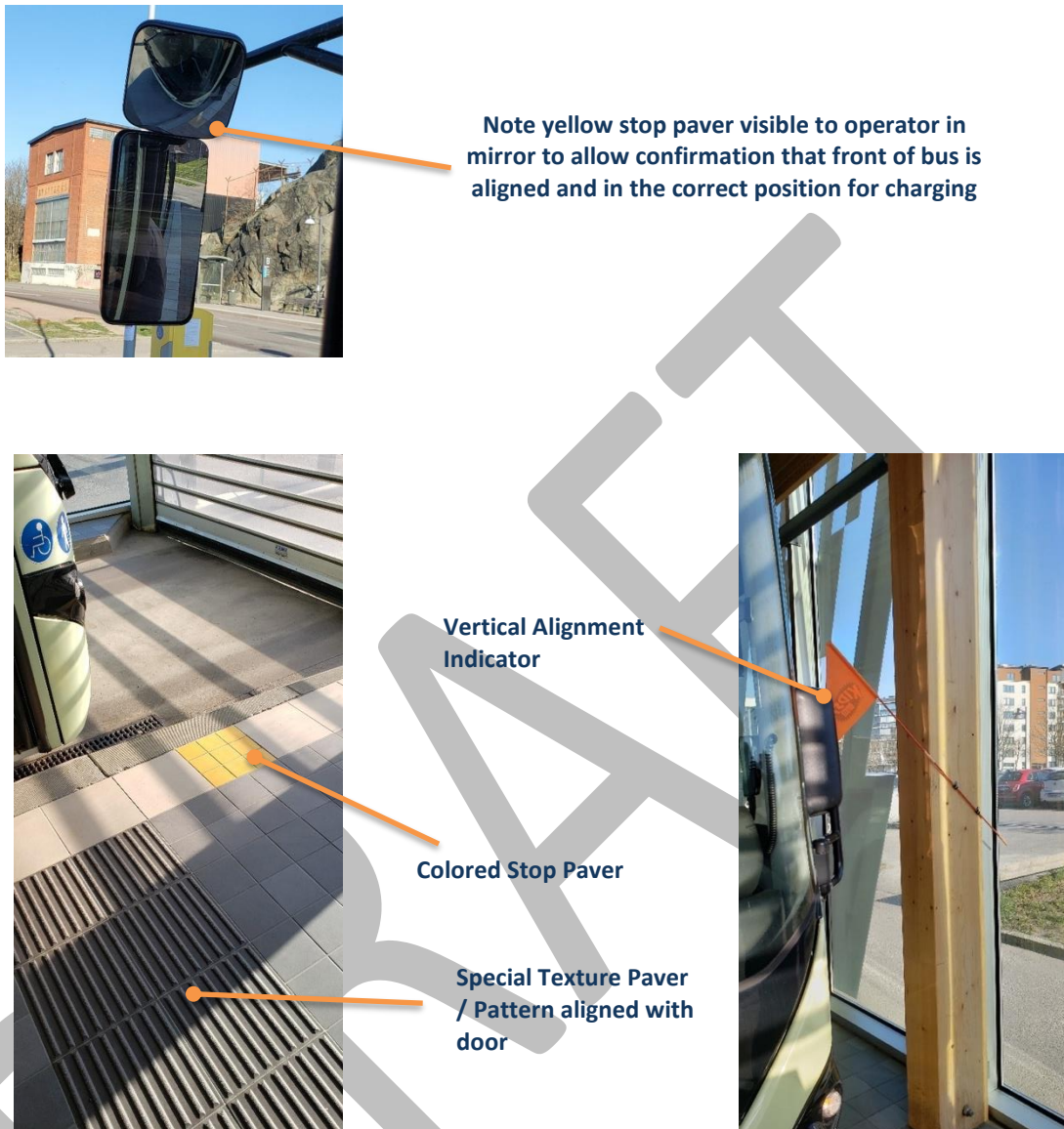
Figure 14 - Overhead Charging Visual Stop/Position Indicator Examples
